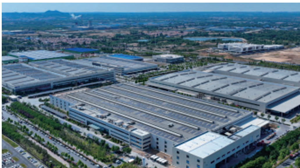
The photo shows Haier Sino-German Ecopark in Qingdao, China, which has become the world's first "lighthouse base" for carbon neutrality.
