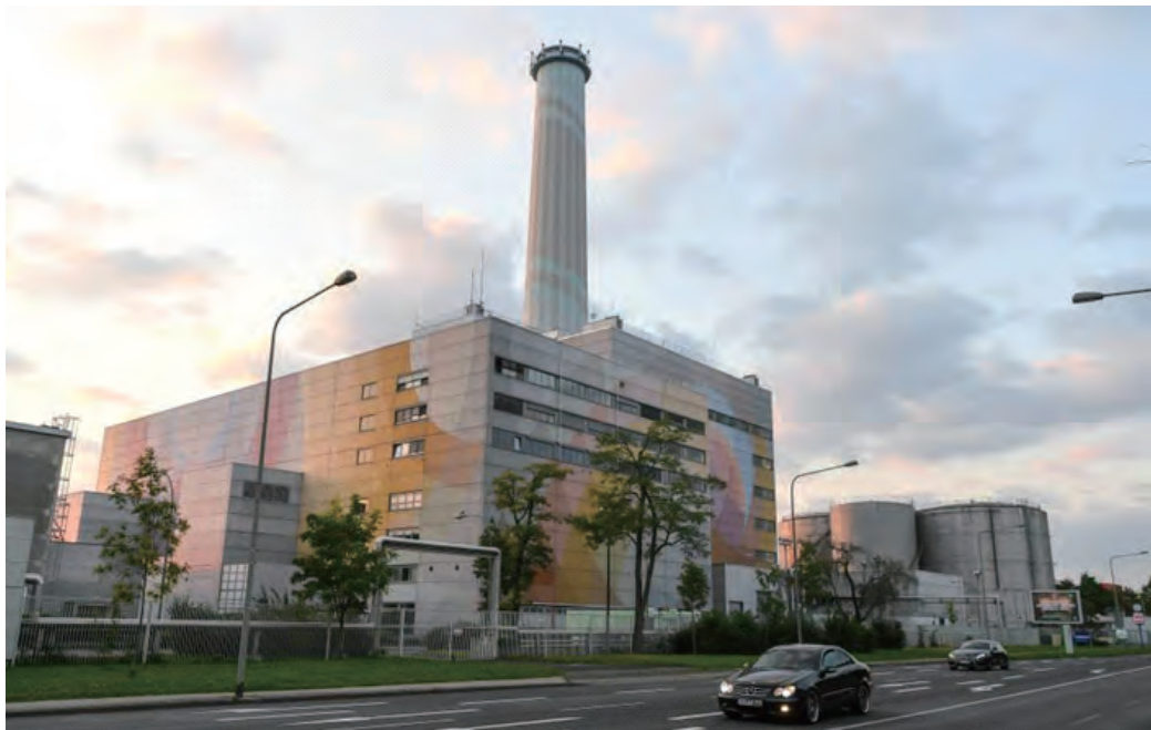
A thermal power station photographed in Frankfurt, Germany in October 2021.
