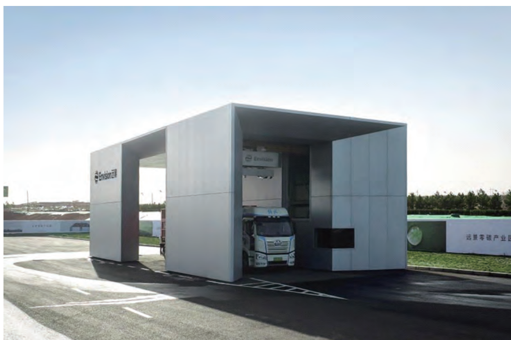
At the Envision AESC Ordos Zero-Carbon Industrial Park, the battery of a heavy truck is being swapped.
